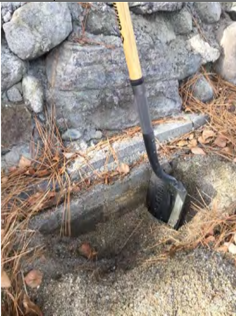
Photo 7: Concrete footing of rock wall
