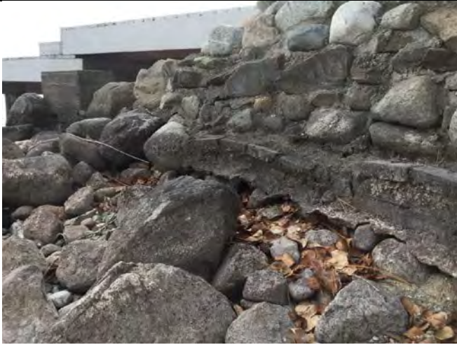
Photo 5: View of scour along base of rock wall footing (poured concrete)
