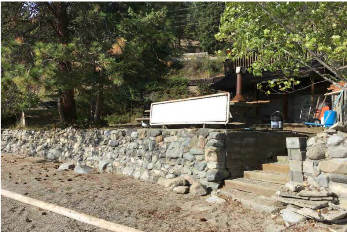
Photo 4. View looking southwest of foreshore modifications (retaining wall and stairs to foreshore) within the subject property.
