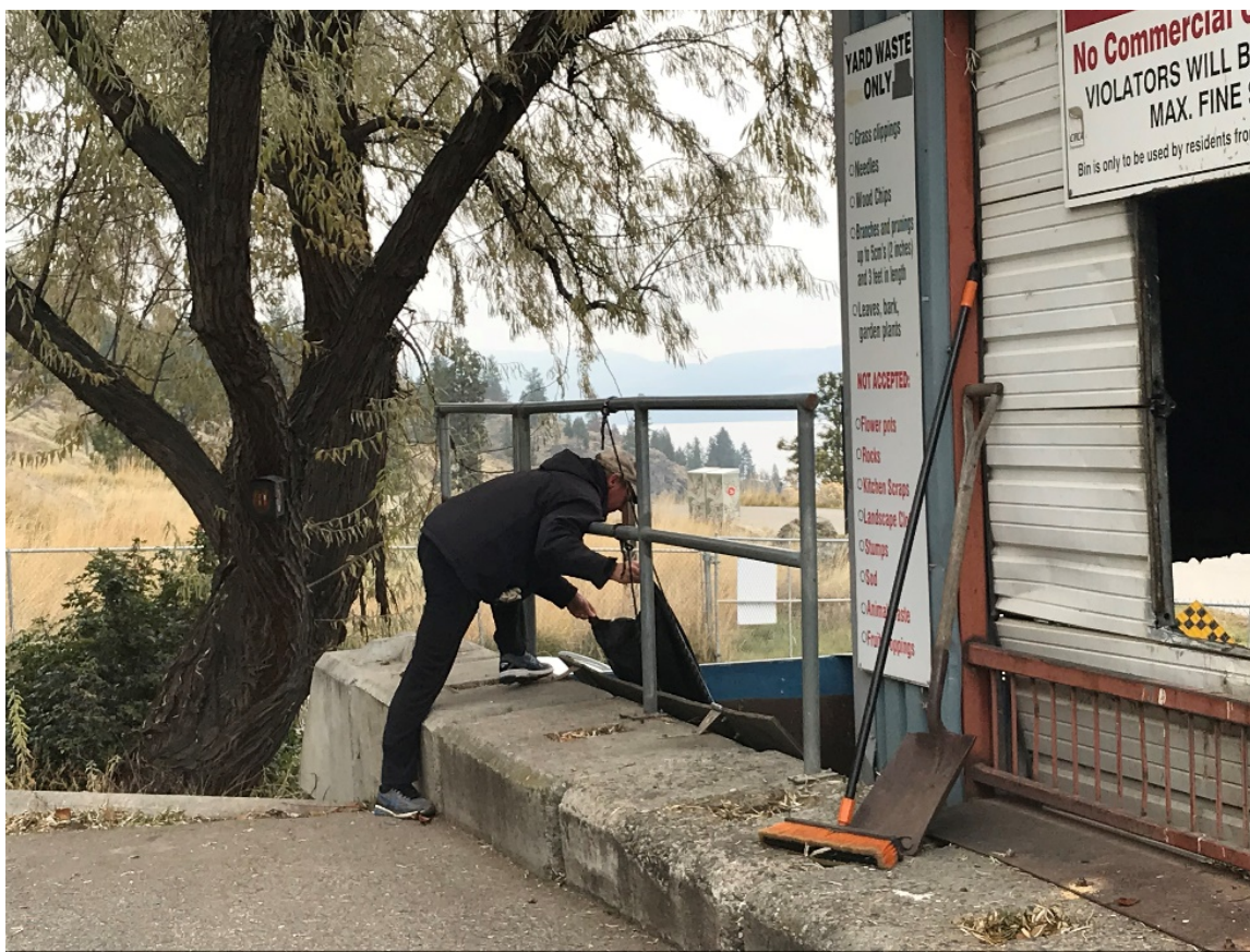
Figure 3 Hazardous retaining wall where user is required to step down from yard waste drop-off area.
