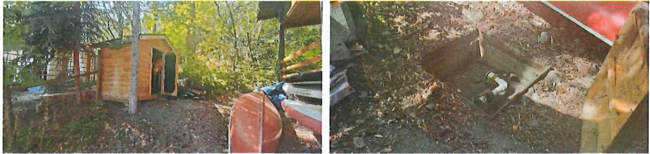
Photo 7 – Storage shed over septic tank and pump
