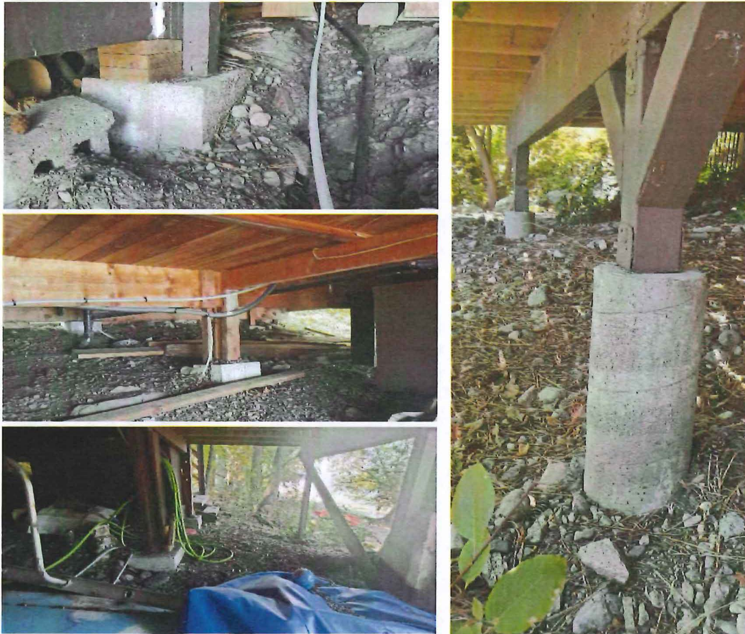
Photo 6 – Shallow concrete footings on Sands and Gravels
