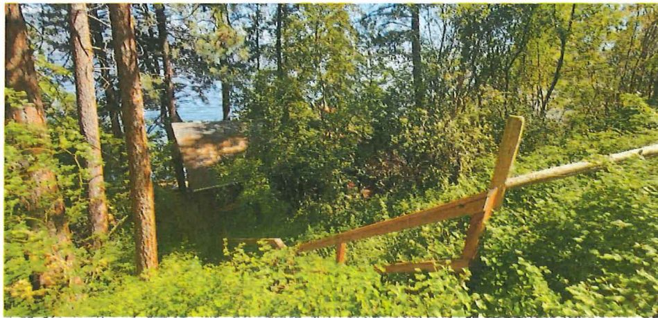
Photo 8 – Vegetated slope behind the cabin, below access road
