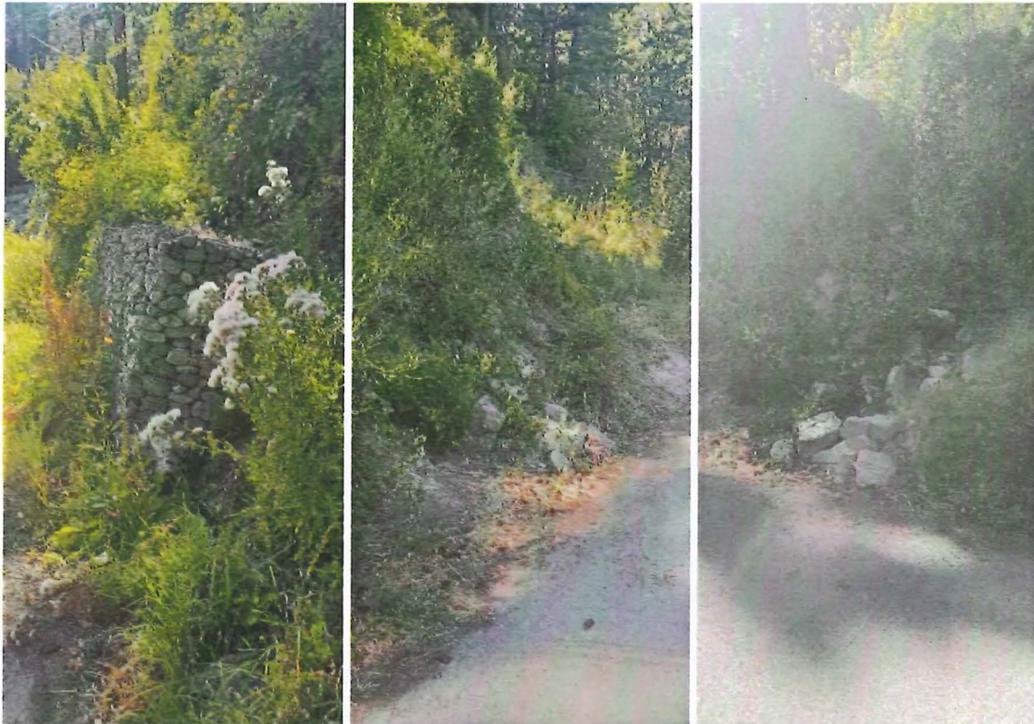
Photo 9 – Forested slope above access road, groundwater seep and bedrock outcrops
