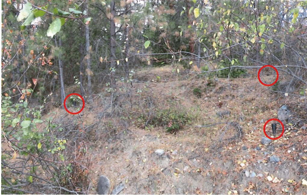
Photo 3: Looking west and uphill from near the bottom of part of the leaching field. Dug terraces are visible along with black PVC pipe (circled in red). (Date of Photo – September 19, 2017).
