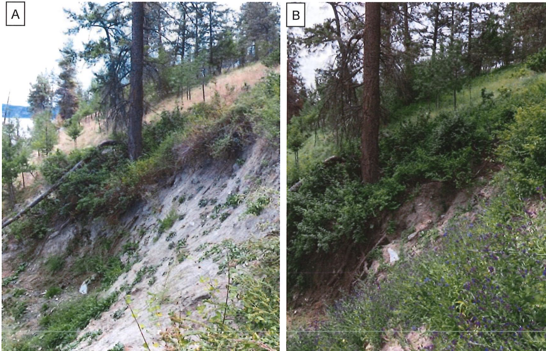
Photo 7: Looking south along the main backscarp of landslide 2. A) September 19, 2017. B) June 29, 2018.
