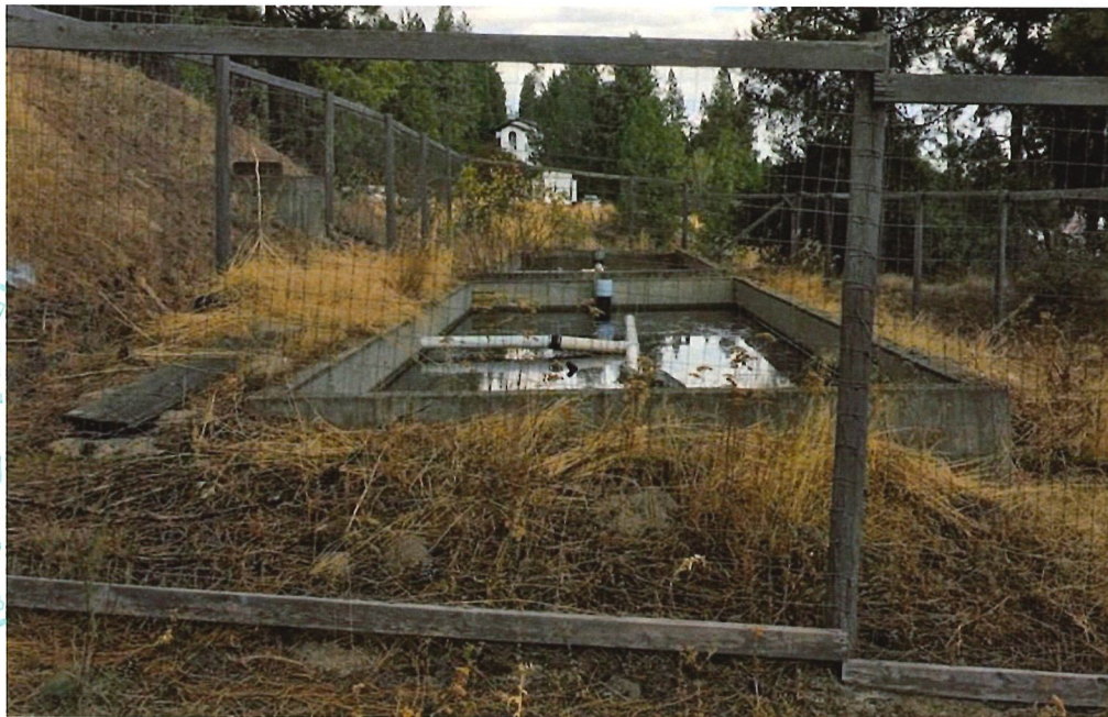
Photo 2: Looking north across the existing sand filters. (Date of Photo – September 19, 2017).
