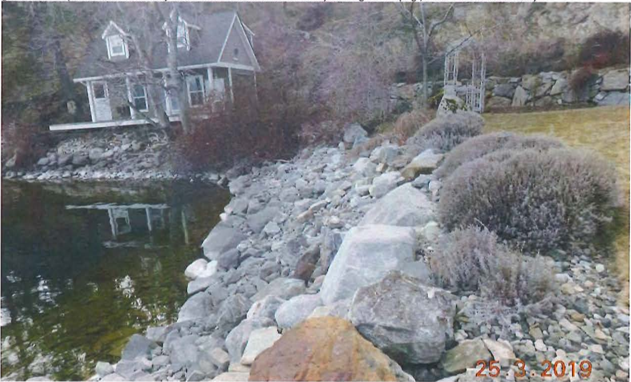
Photo 8. After fill is removed, the shoreline will match the natural shoreline that can be seen fronting the cabin in the left of the photo. Native shrubs and trees will be planted to restore the area to native ecosystem condition.
