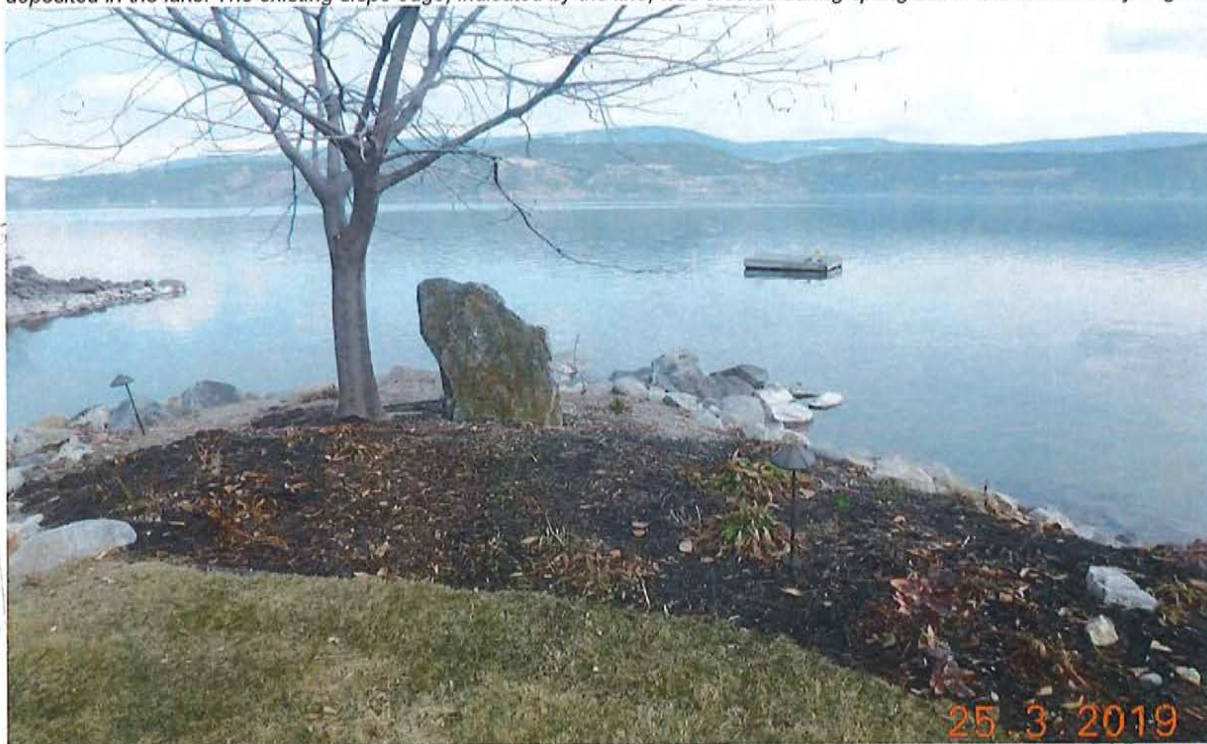
Photo 6. The existing rock groyne, with tree, will be retained so that existing Kokanee spawning habitat is not lost. The groyne will effectively become an island at high water levels. Native trees that are adapted to water will be planted on the island.
