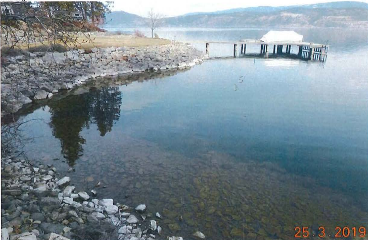
Photo 10. The fill area will become a series of flood benches that will vary from being underwater at all times to only being flooded during extreme events (like that seen during spring 2017). There will be a net habitat improvement.
