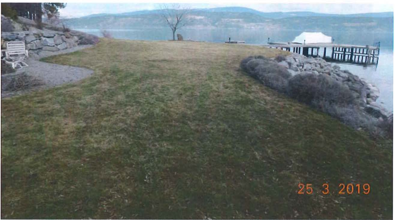
Photo 12. Areas above the average lake level of 342.15 m will be naturalized with large woody debris, large rocks (picked from the existing rip-rap), and native plants that are suitable to the flood regime. See detailed grading plan.
