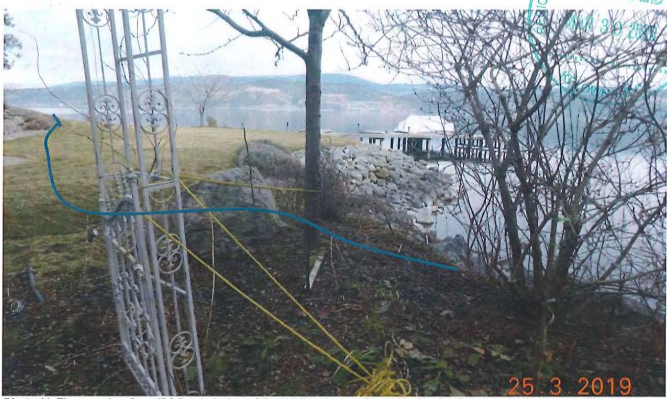
Photo 11. The new shoreline will follow trajectory of the existing shore to the south. See line for approximate example. The area to the right of the line will be a series of four flood benches and a Kokanee spawning bench.
