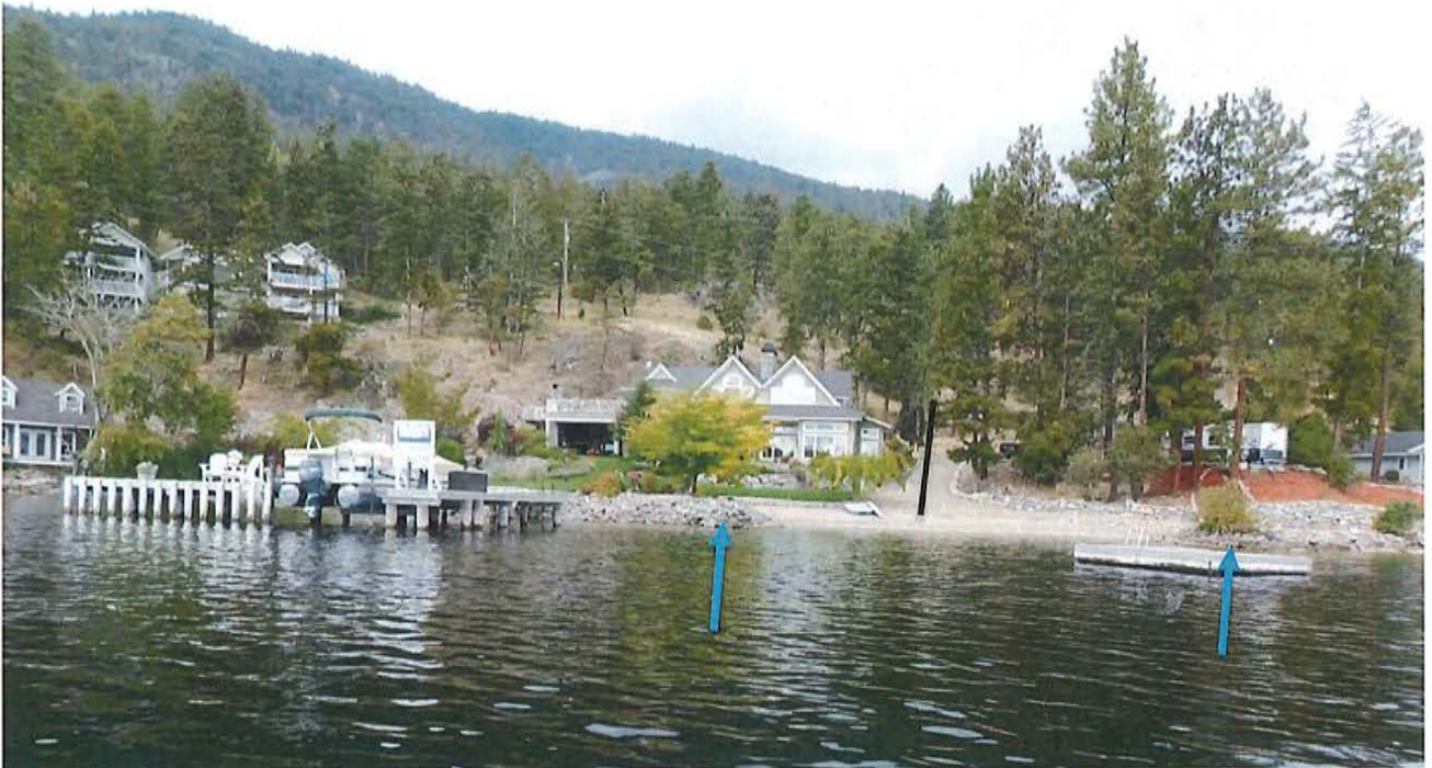
Photo 1. 2677 Westside Road is the property on the left side of the picture. Black line is approximate property boundary. There are two rock groynes marked in the Foreshore Inventory Mapping database, and indicated by arrows.
