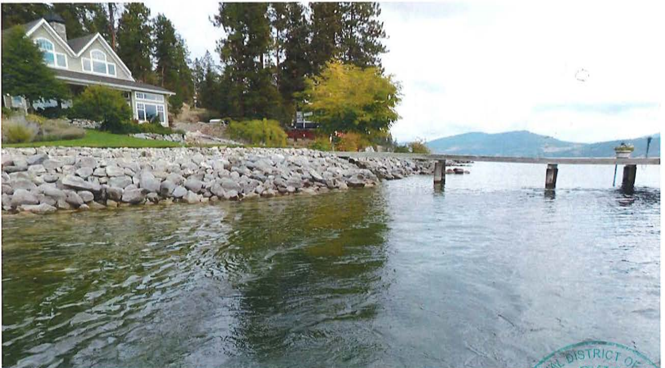
Photo 2. Fill area and dock at 2677 Westside Road. The plan is to remove some of the fill and create flood benches to enhance fish and wildlife habitat.
