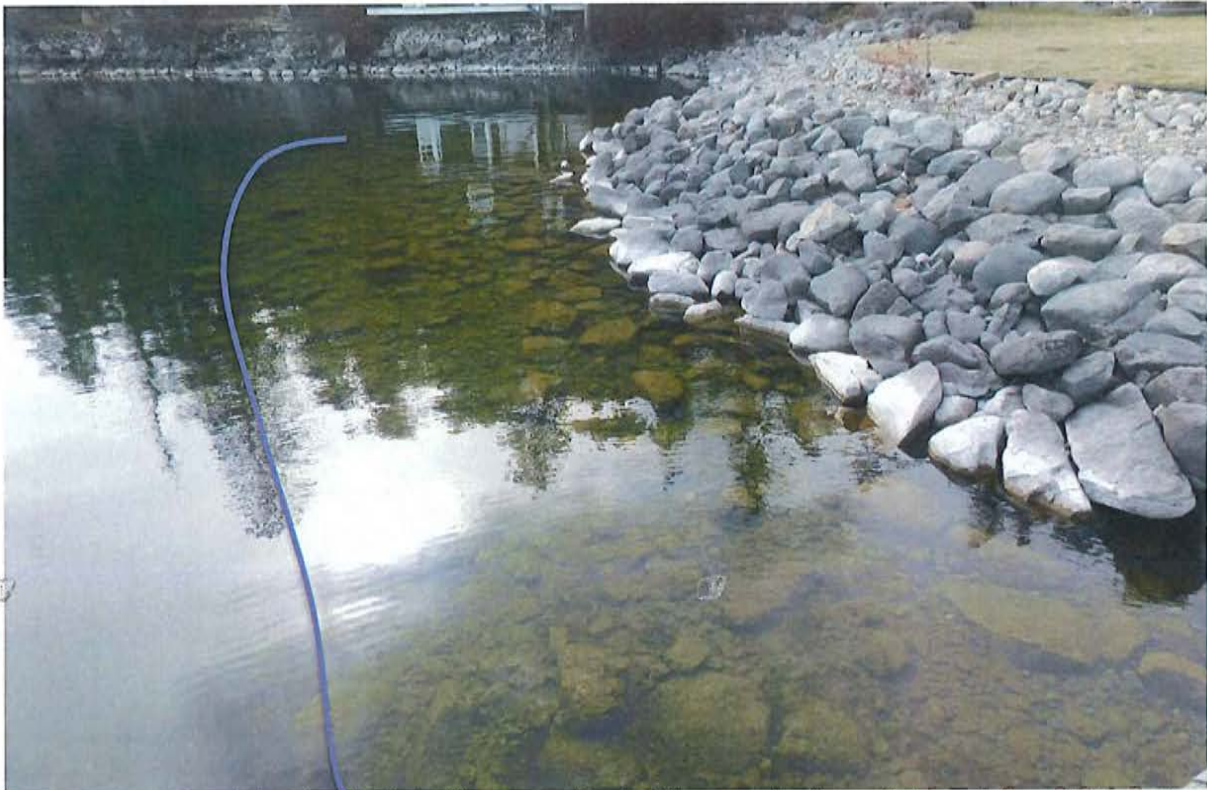
Photo 5. View of the existing shoreline that will be removed to about the same elevation as that seen in the water to create a 10 to 15 m wide Kokanee spawning shelf, expanding on the size of the shelf that can be seen in the photo. No materials will need to be deposited in the lake. The existing slope edge, indicated by the line, was created during spring 2007. It is anchored by large rocks.
