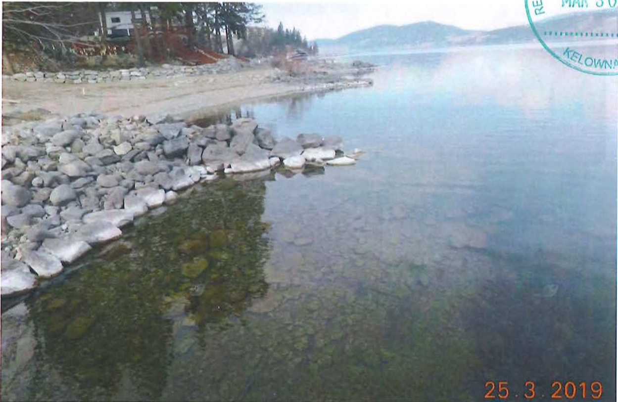
Photo 7. This photo shows the high value Kokanee spawning habitat that has been retained by the rock groyne. Similar-size gravel will be placed as is normally found in Black-zone Kokanee spawning areas (e.g., Paul's Tomb shoreline).
