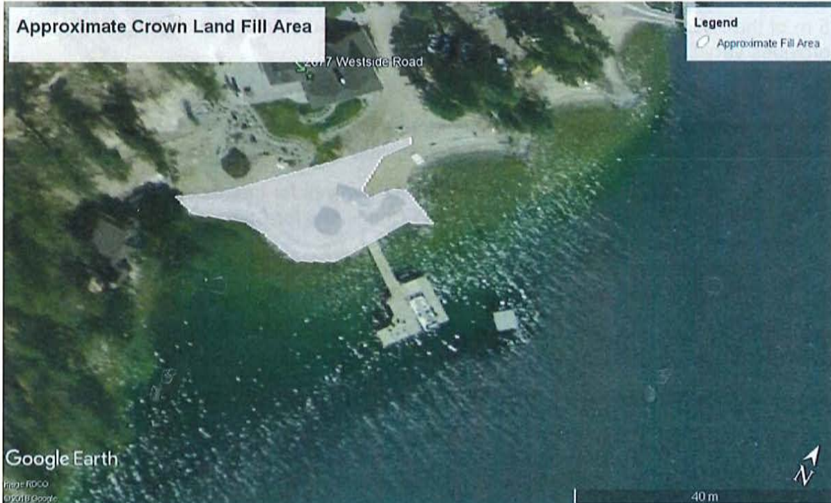
Photo 1. View of the approximate fill area in the lake fronting 2677 Westside Road. The dock and shoreline remain virtually unchanged in 2019 as seen in the air photo.
