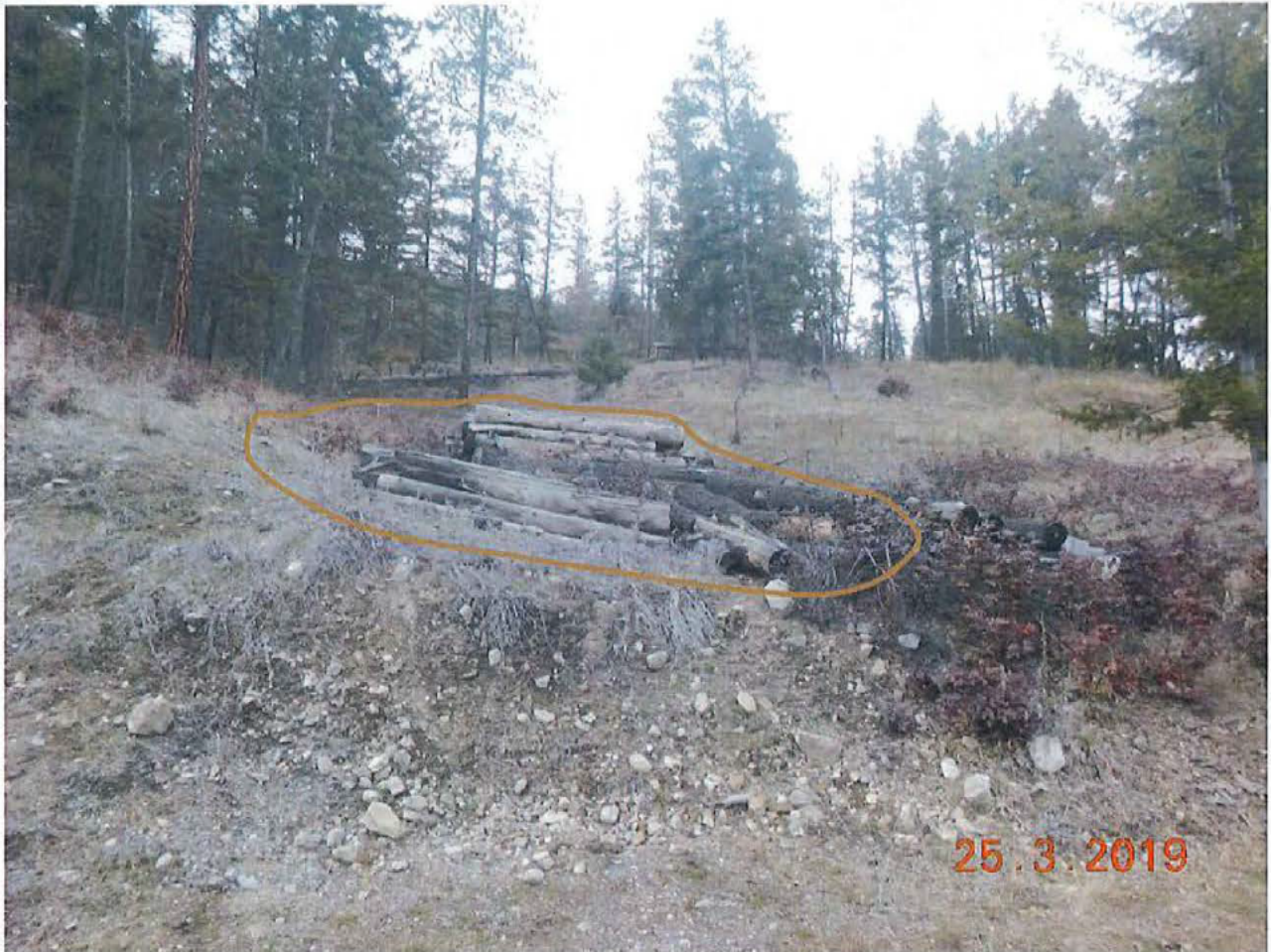
Proposed fill placement location shown in orange polygon. Logs will be removed, top soil stripped, and these materials will be used to reclaim the site after fill placement.
