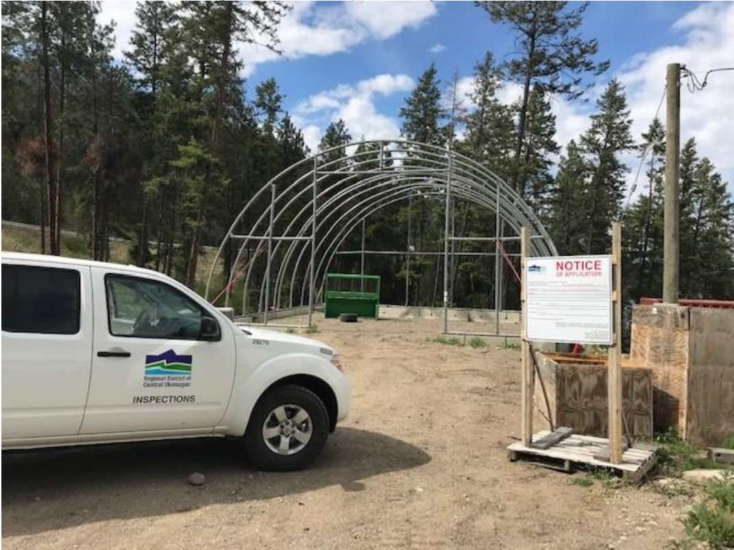
Image of Accessory Building from Denison Road
