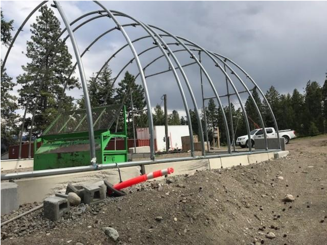
Image of Accessory Building towards Denison Road
