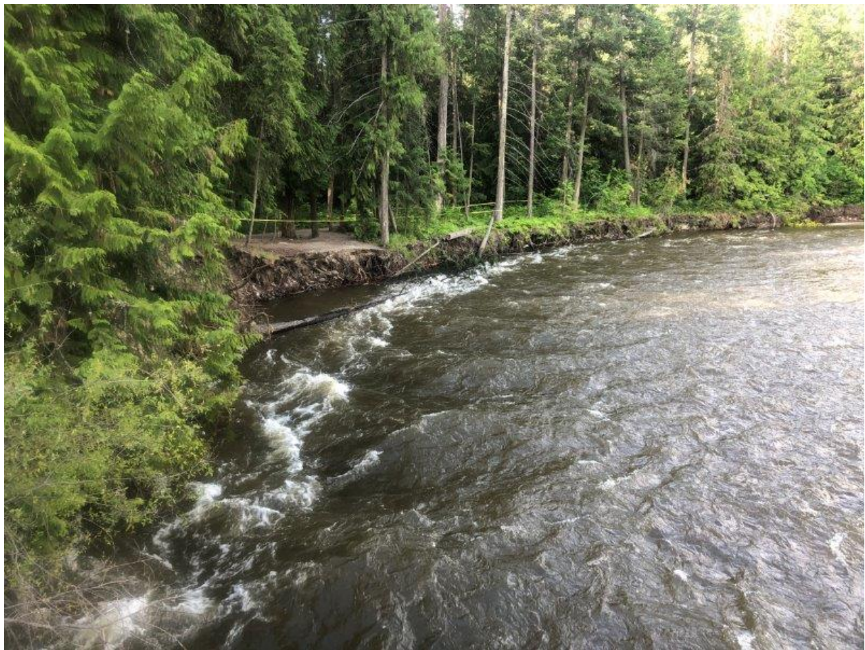
Photo 2 – View looking upstream from bridge at right abutment
