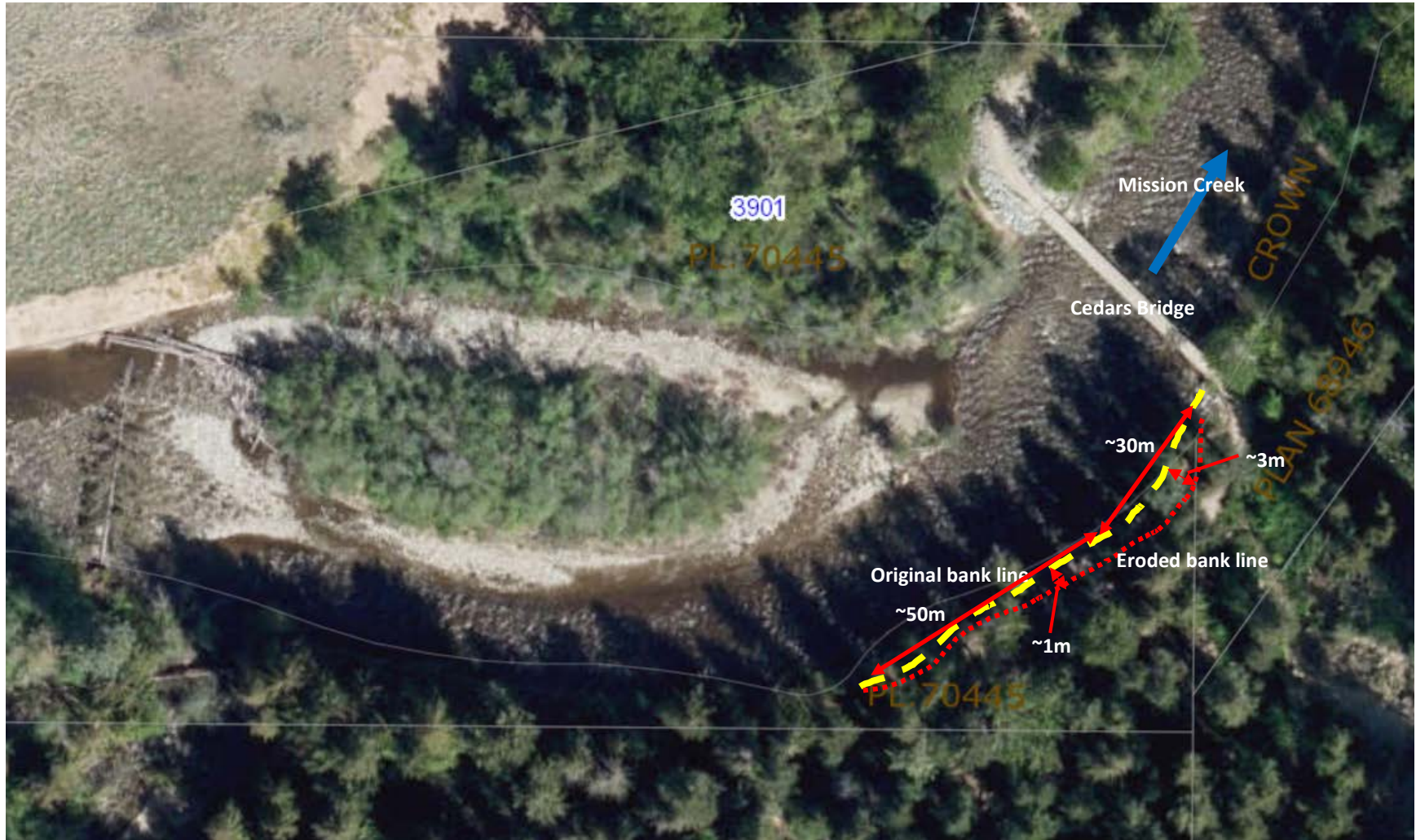
Figure 2 – Mission Creek at Cedars Creek Bridge 2020 erosion
