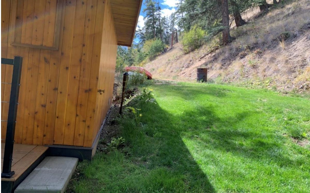
Photo 5. Sauna Structure on left. Proposed Sauna location will be nearer to the barrel pictured. Note steep nature of the mid-seral forest in background.
