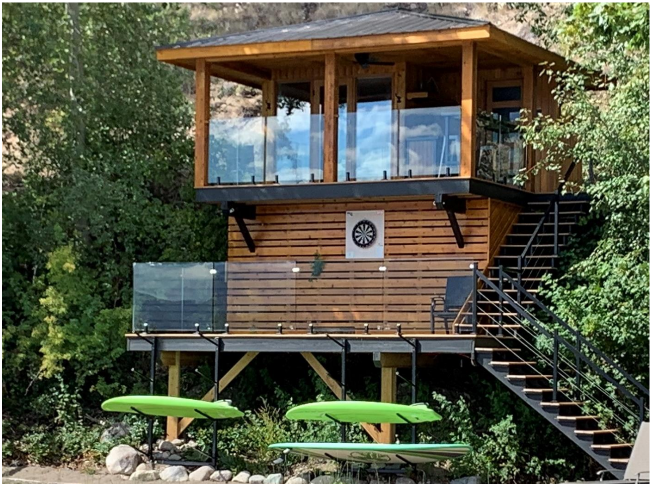
Photo 1. View of the Sauna that encroaches into the Habitat. The Sauna Structure will be removed and placed >15 m from the Present Natural Boundary. Vegetation is growing out of the space below the sauna. The stairs will remain to provide beach access from the relocated sauna.
