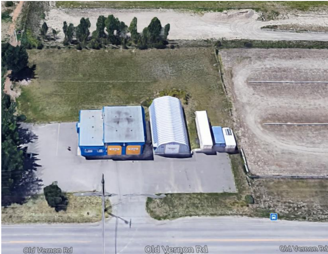
Figure 2:5: COSAR Buildings Oblique View
