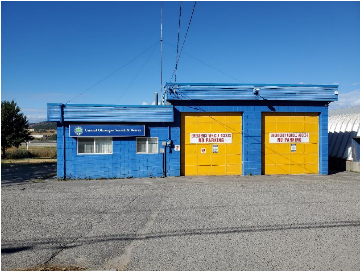
Figure 2:7: Main High Bay Building
