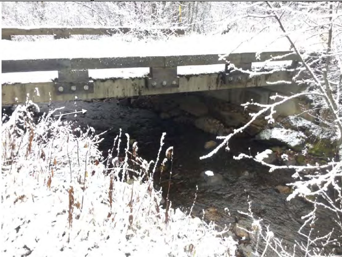
Photo 11: Whiteman Creek – Bridge at South Whiteman Creek (South Fork)
