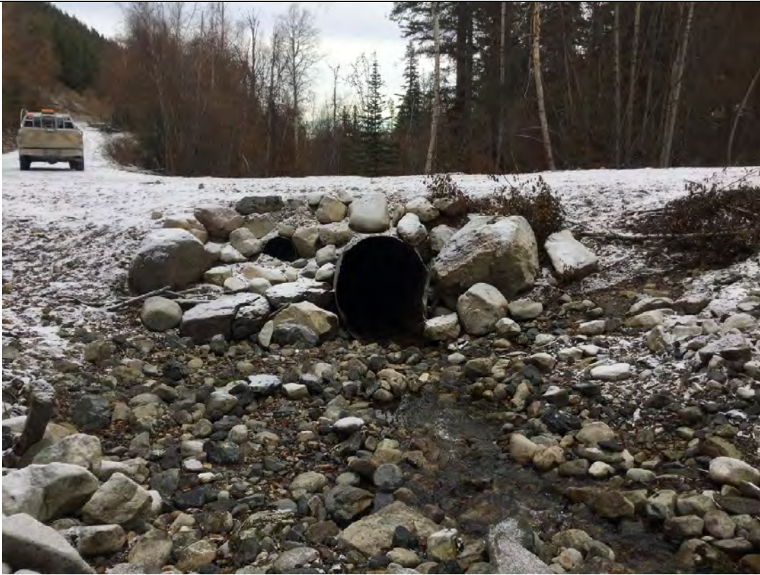
Photo 16: South Whiteman Creek, culvert along South Fork FSR
