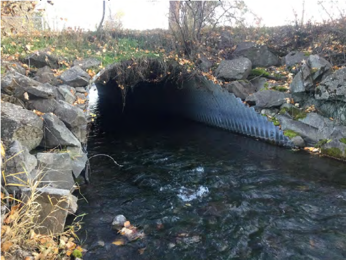
Photo 14: Equesis Creek arch culvert at Westside Road, view downstream
