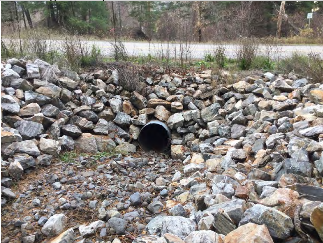
Photo 8: Newport Creek at Westside Road
