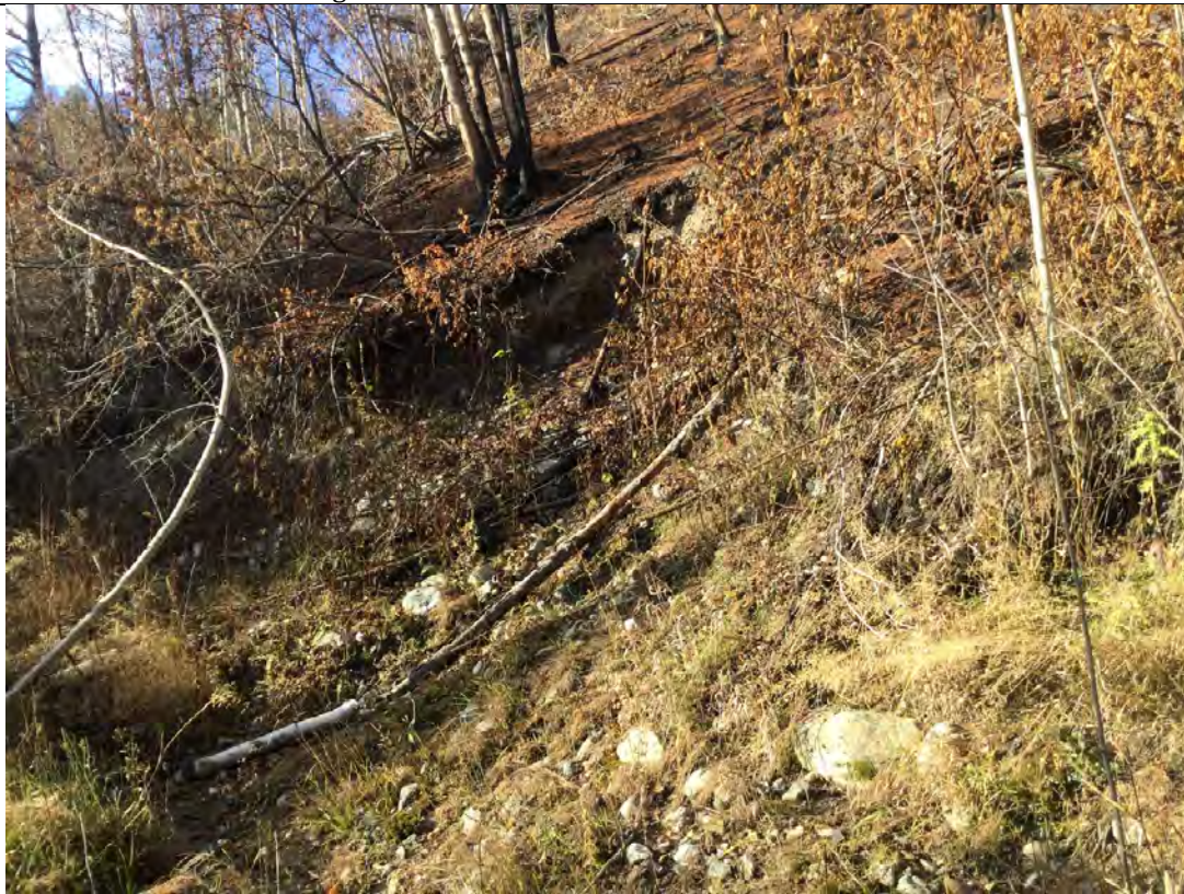
Photo 6: Observed slope instability (headscarp and tension cracks) near the Gates Creek crossing on Siwash Creek Road (part of the larger Nashito Slide)
