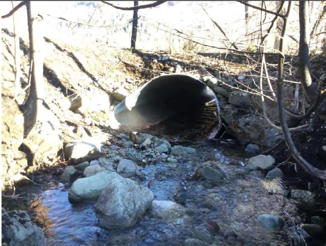
Photo 8: McGregor Creek culvert at FSR Crossing, view downstream
