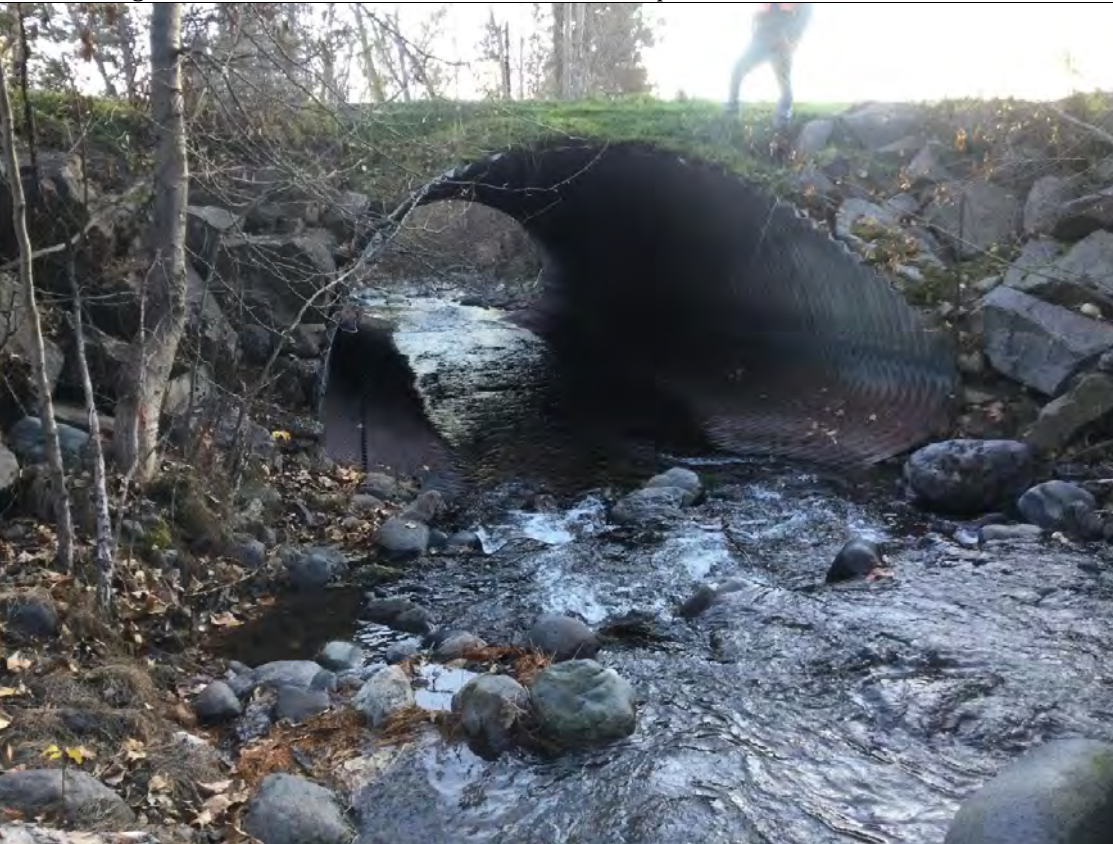
Photo 8: Naswhito Creek arch culvert at Westside Road, view downstream.
