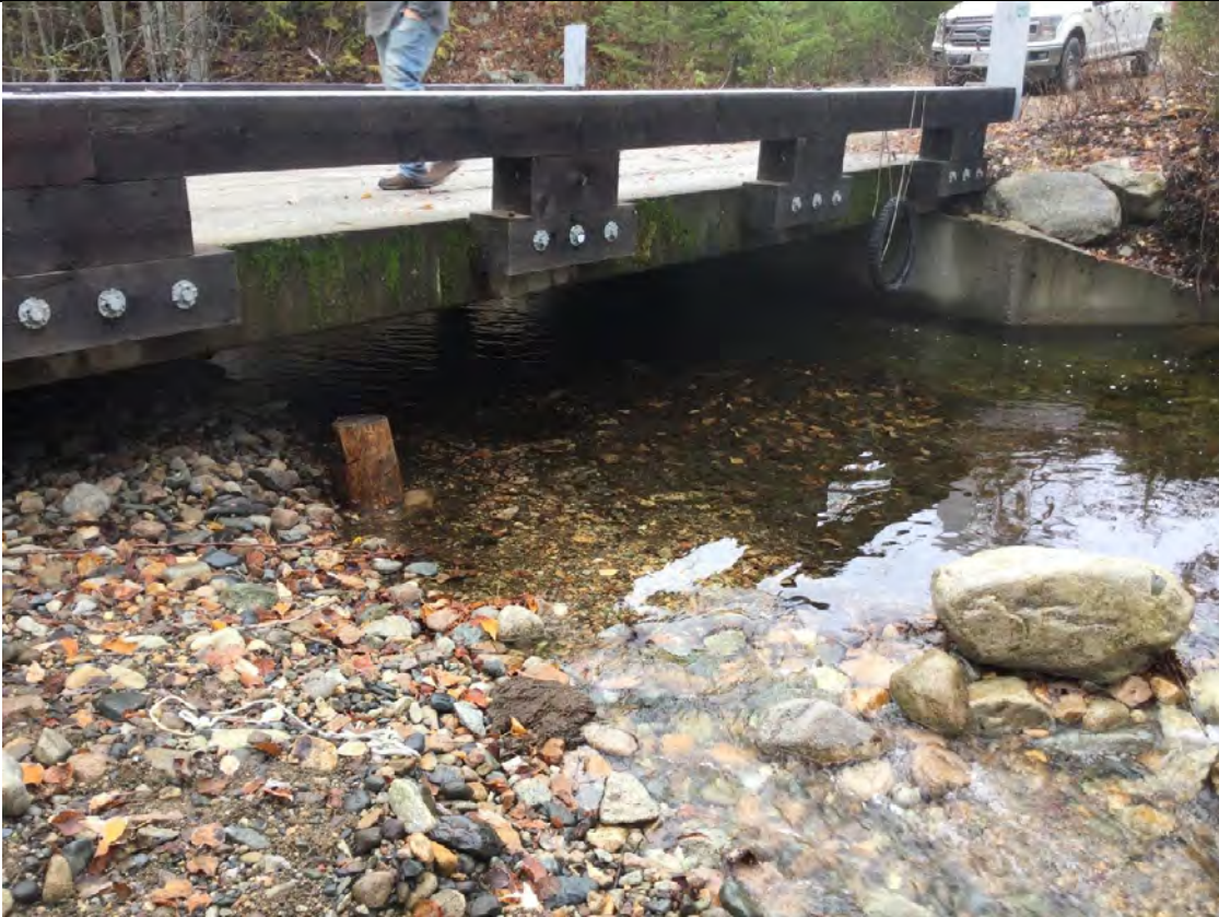
Photo 12: Whiteman Creek - Bridge at Maw FSR
