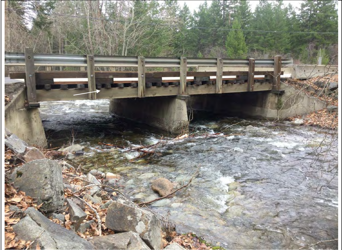
Photo 7: Whiteman Creek at Westside Road (concrete bridge ~10m span)
