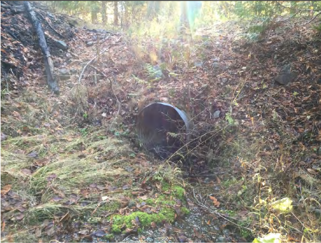
Photo 5: Gates Creek culvert crossing on Siwash Creek Road
