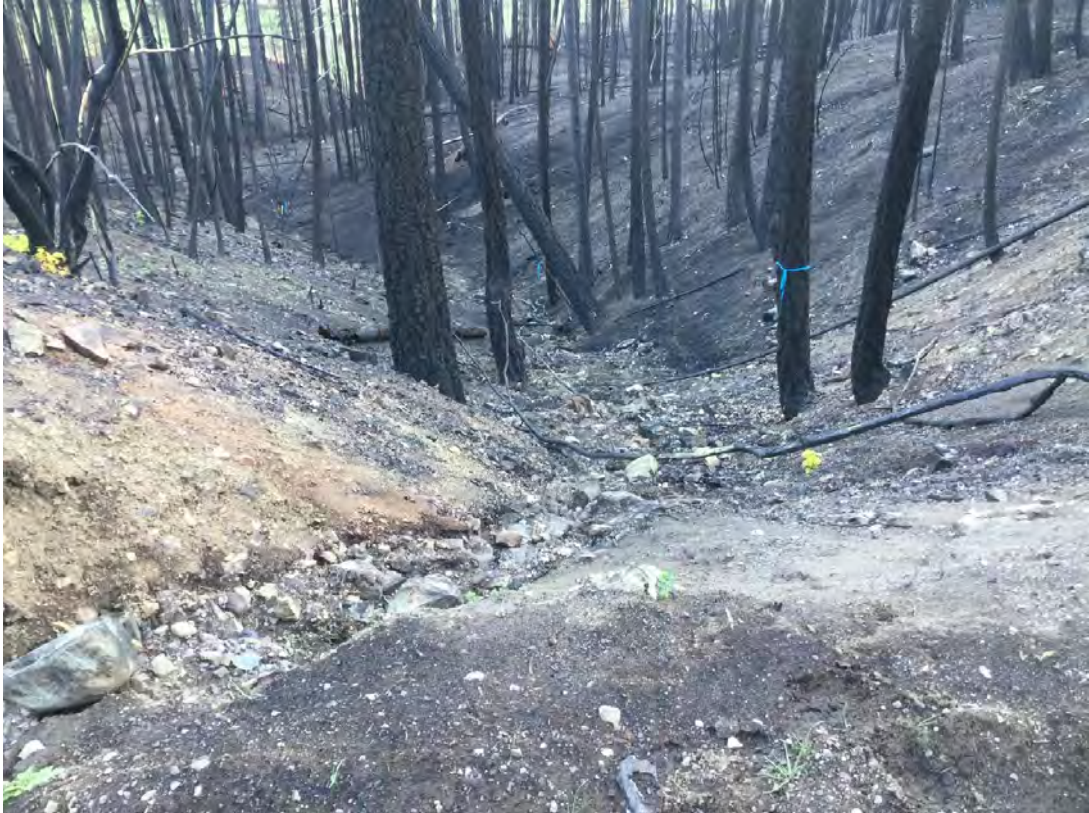
Photo 2: Face Unit south of Naswhito Creek, burned gully below access trail, view downslope towards Westside Rd.
