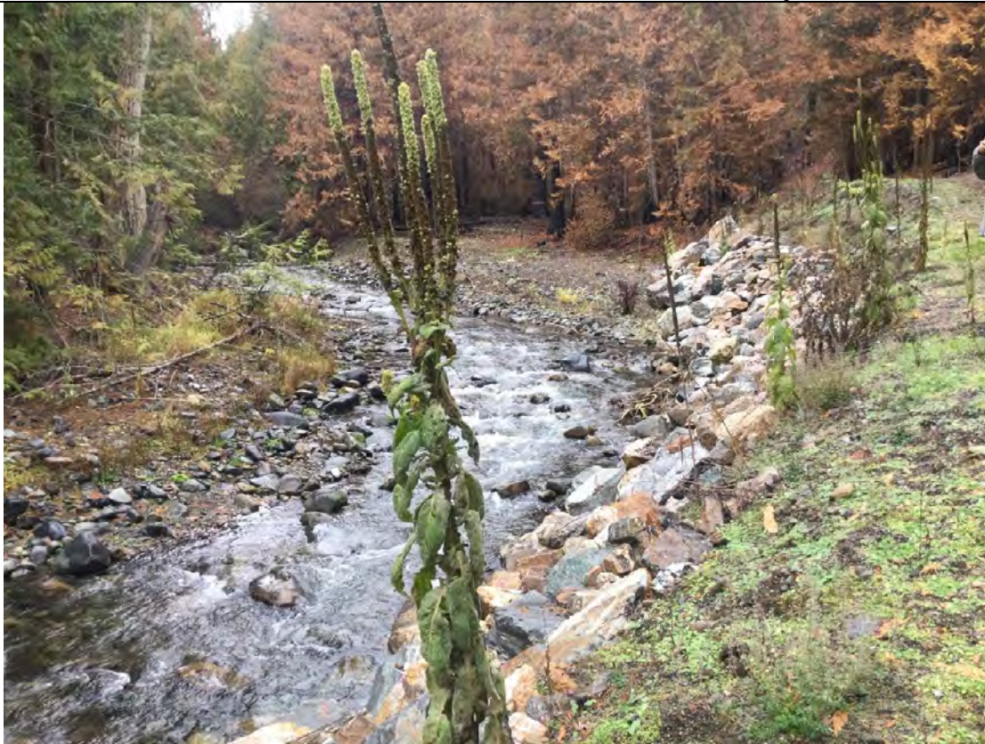
Photo 11: Lower Equesis Creek riprap armour along left bank, view upstream.
