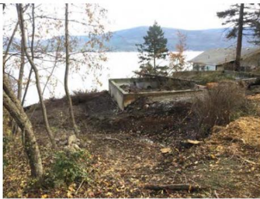
Photo 1: View of upper part of lot at 37 Nerie Rd, culvert outlet and stream flow in foreground
