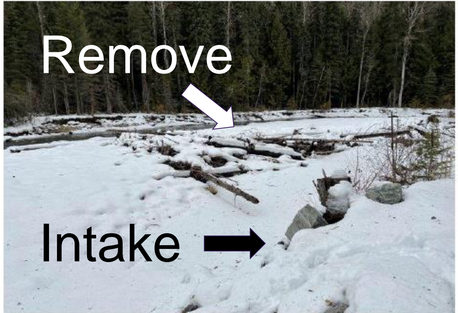
Phot 3 – Wood debris accumulations on the bar at the intake.
