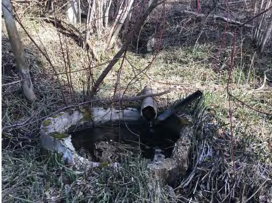
Photo 11. View of remnant catch basin associated with Rockface Creek tributary.
