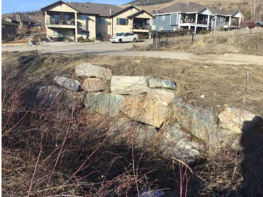
Photo 17. View of suspected culvert requirement along the eastern subject properties' boundary over Rockface Creek.
