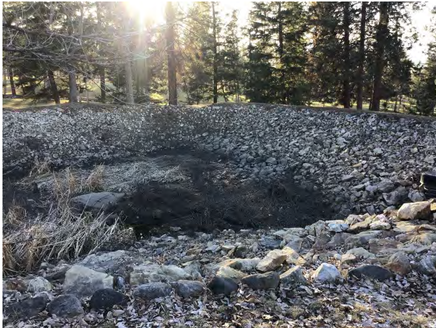
Photo 20. View looking at catch basin likely associated with Rockface Creek and its tributary just north of the northwestern subject properties' boundary.
