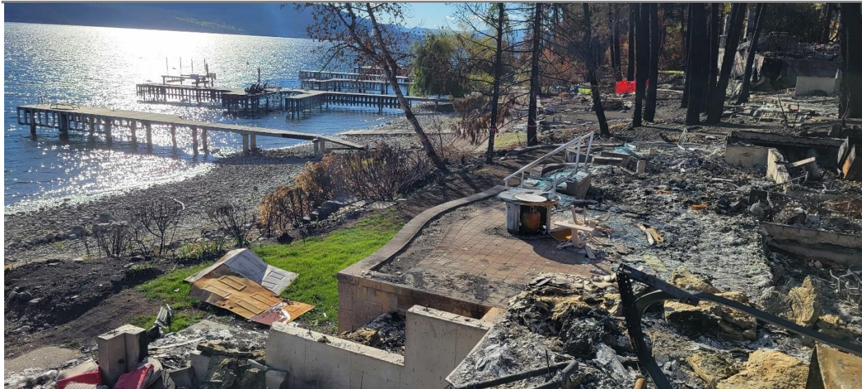
Photo 1: Riparian portion of the Site, post-fire and pre-demolition, patio for retention in the foreground, gardens for retention in the background behind the stair rail 211006
