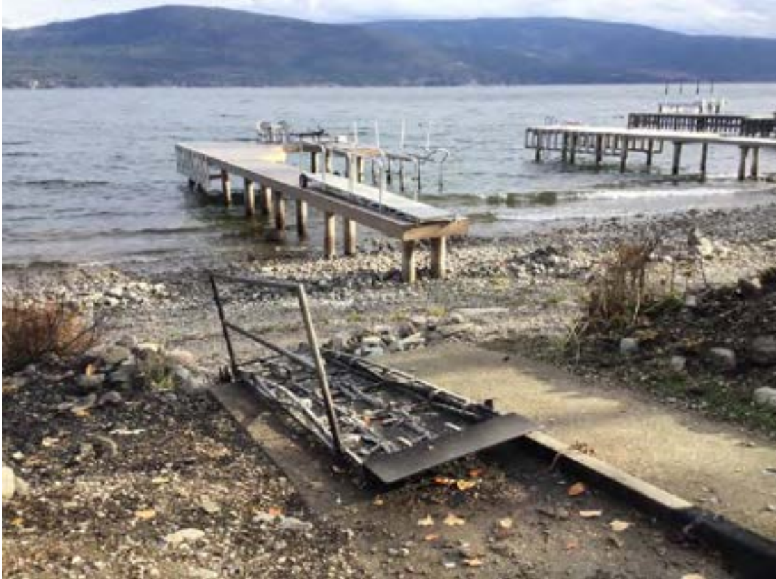
Photo 1: View of foreshore area at 7 Nerie Rd.
