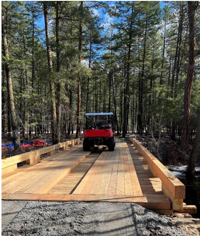
Trepanier Creek and new bridge crossing.
