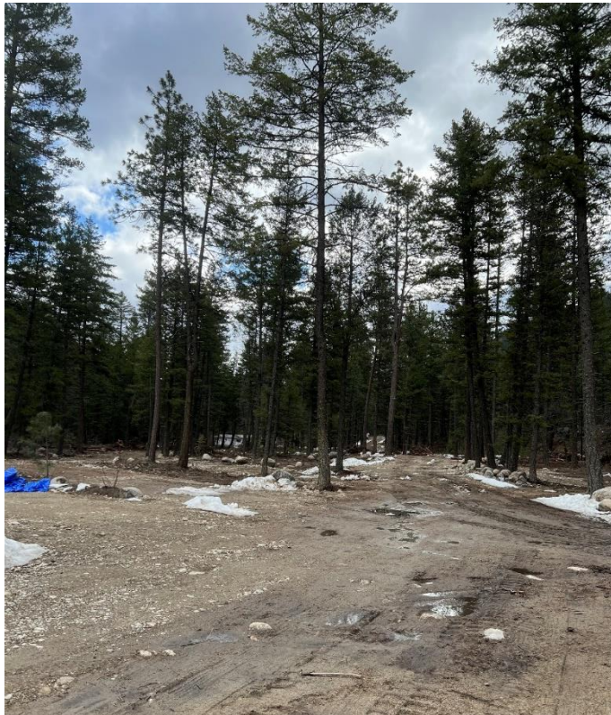
Photos of the campground under construction.
