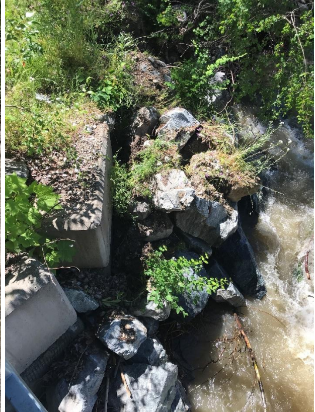
Failing Abutment Protection – June 22, 2022
