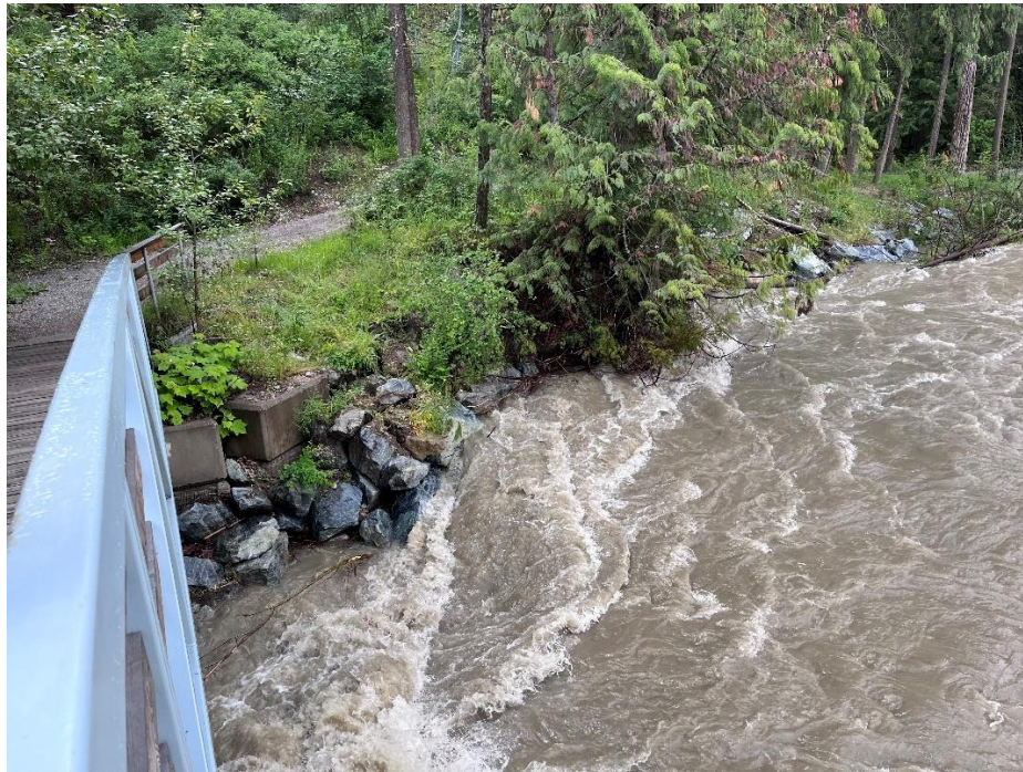
Scour Behind Cut Off Wall – Failing Abutment Protection
