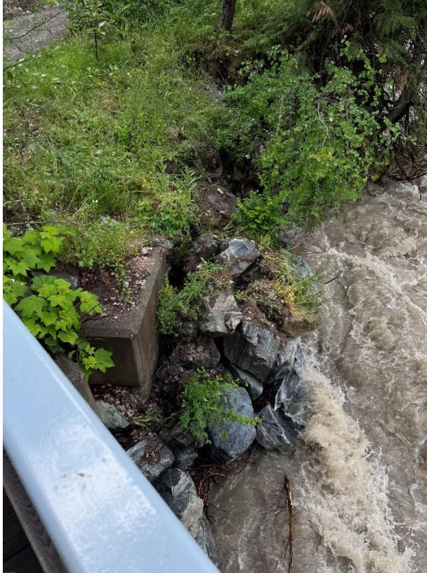
Failing Abutment Protection – June 20, 2002
