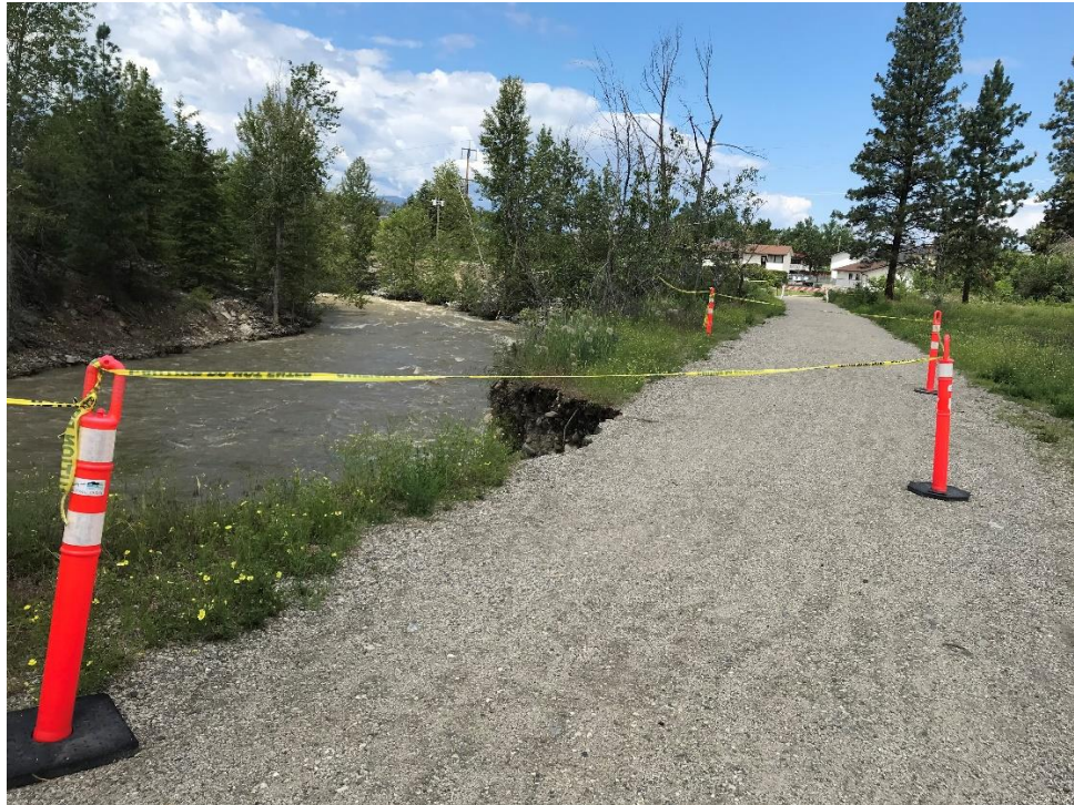
Pasadena Section Looking Downstream – Loss of Trail / Bank Scour – June 20, 2022
